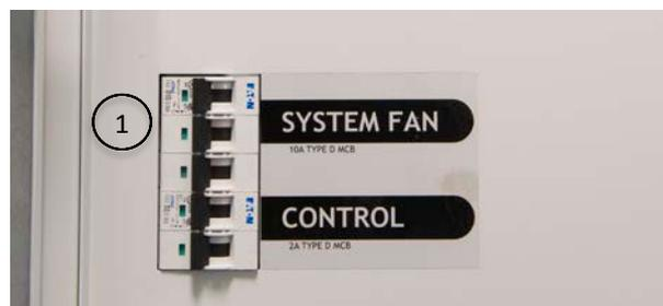
**Figure 5: Fan circuit MCB**
