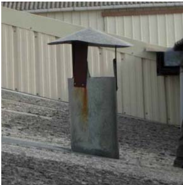
Figure 14: Examples of unacceptable ducting installations
