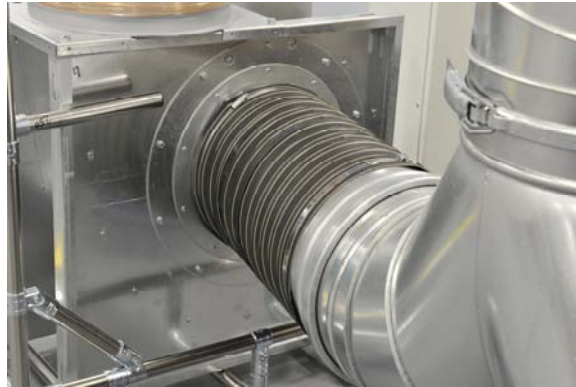
Figure 8: Cooling fan connection to ducting run
