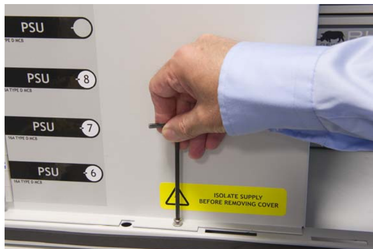
Figure 11: Removing the inner panel
