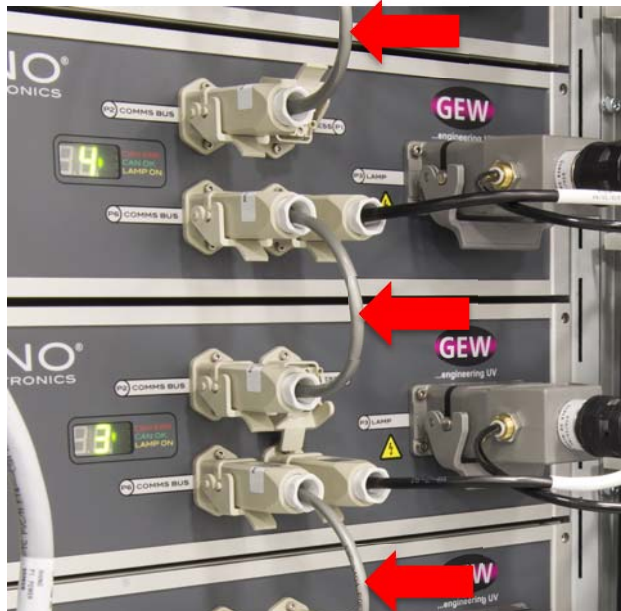
Figure 18: CAN Bus connections between adjacent RPSUs
